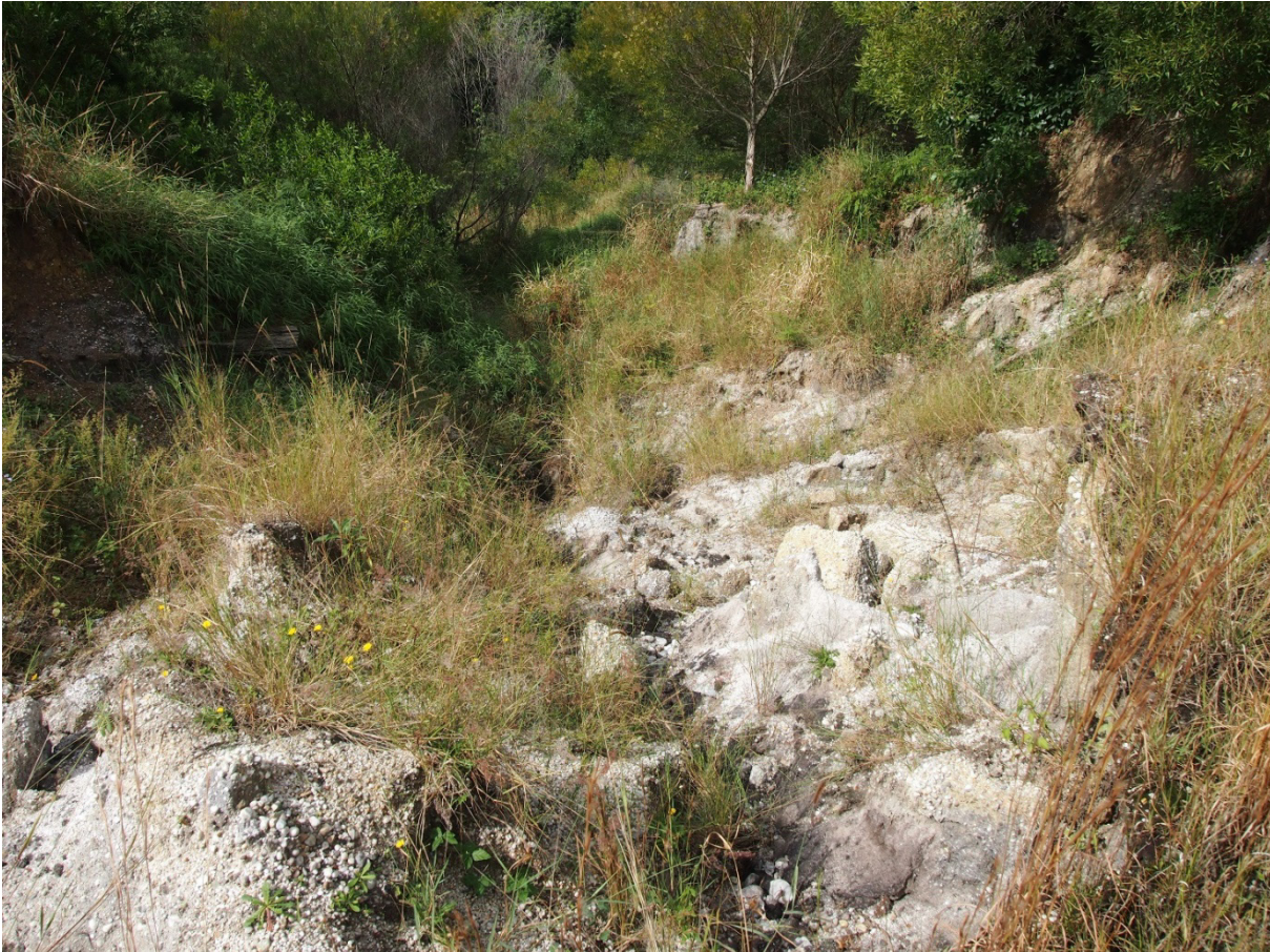
Plate 2: Erosion gully on proposed residential land at top of site
