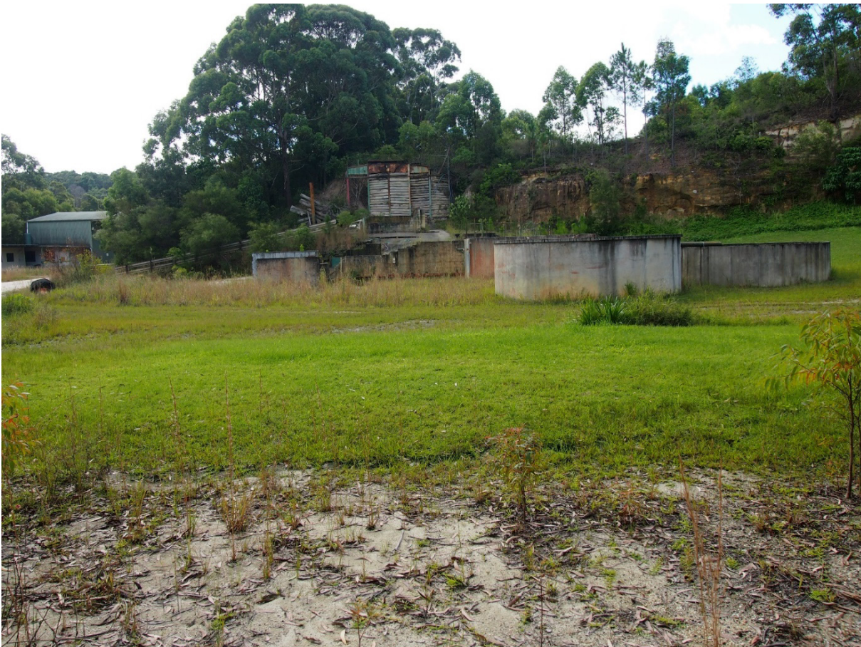
Plate 4: Parts of the site proposed for residential development have a past use that may have caused land contamination
